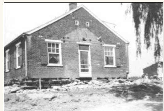
Pictured above is the Lexington school at 811 Furnace Hills Pike in the process of being moved to make way for the new road.
