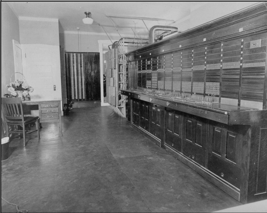
Top: The telephone exchange, one of the locations where Keller worked, located at 136 East Main street (smaller building on right). Left: the interior of 136 East Main street.
