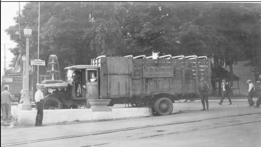
Left: Damages to the fountain in the 1930's were caused by a passing truck.
