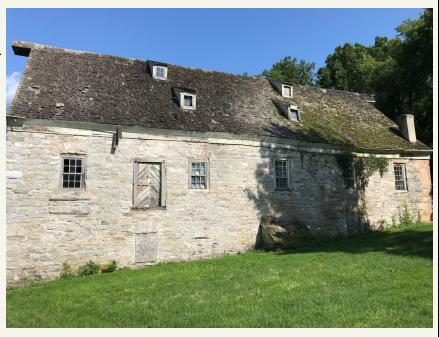
Throughout 1757 Moravians from Litiz and Bethlehem were involved in the tedious construction of not only the new mill but also the mill race extending from Carter Run. Lime stones had to be quarried and used for the base of the mill and the race way. Timber had to be cut from the area and milled in the old, shabby sawmill built several years before.
